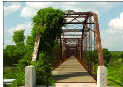
The 1916 Canadian River Wagon Bridge
